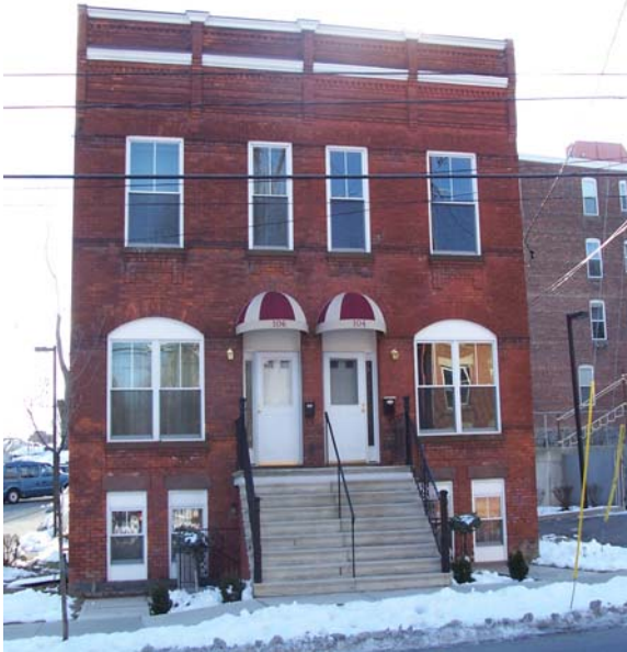
Phase I - 104 & 106 Mansion Street
